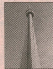
Aliant to Build Communications Tower
