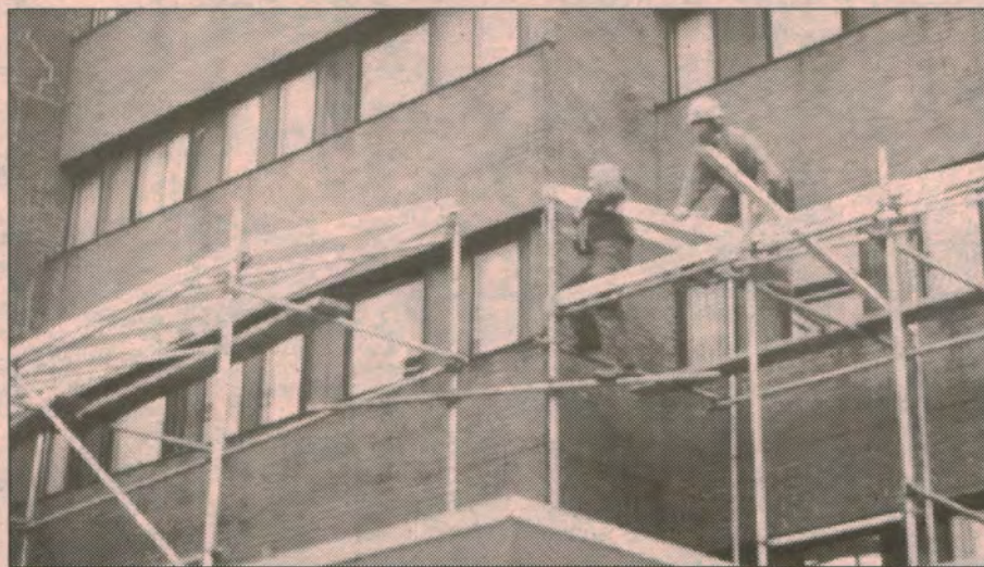
Workers assemble scaffolding as they begin repairs on residence
