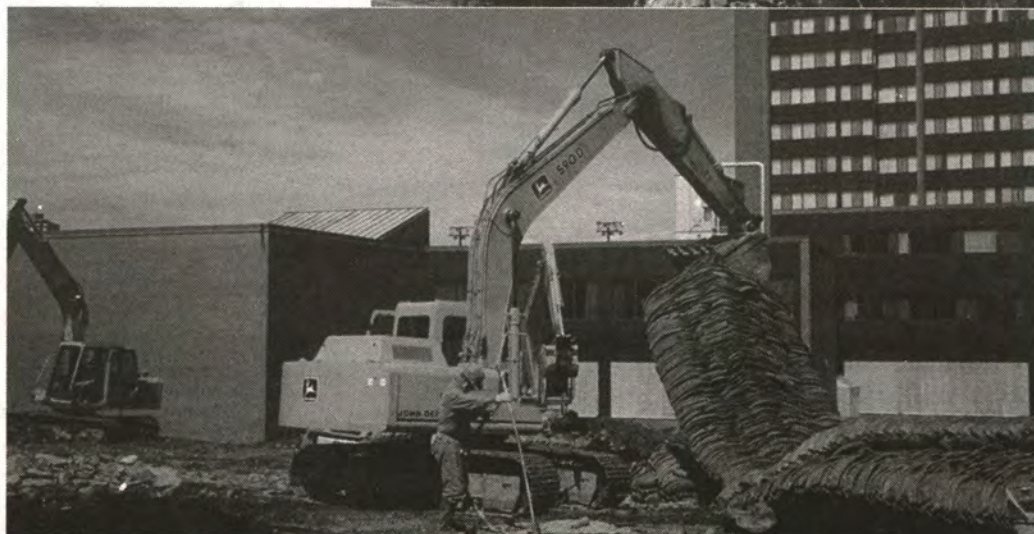
The tire mats are being moved for blasting on June 26.
