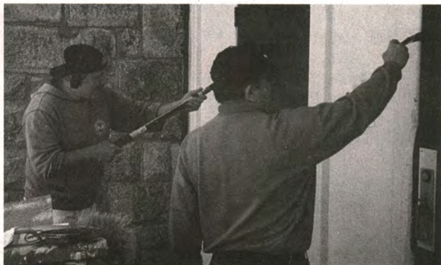
Jim Young and Kenny Slaunwhite, Physical Plant workers, paint over the graffiti at the main entrance of the Alumni Arena.
