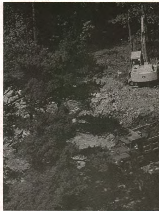
The excavation begins on June 18.
