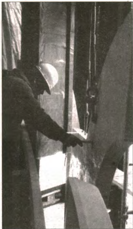
The pre-casting began just a few days ago.
