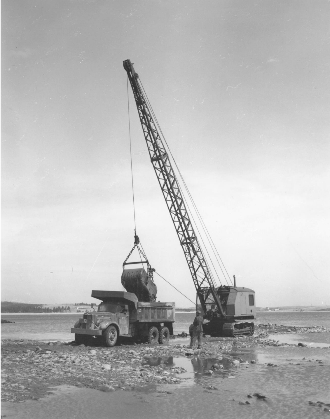
Trynor Construction Company extracting sand and gravel from Silver Sands Beach at mid 20 th century. Courtesy of The Chronicle Herald.
