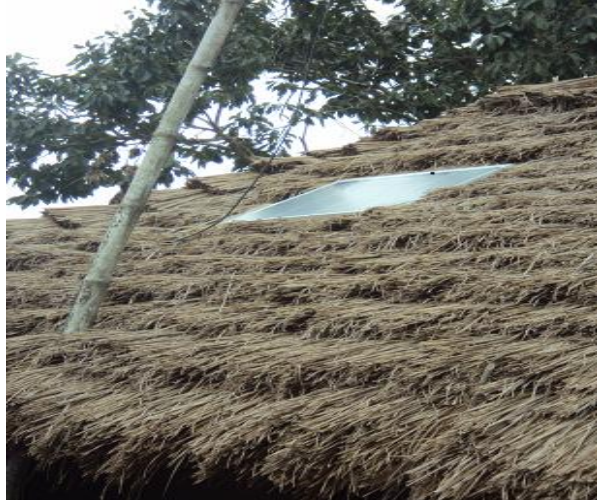
Picture 1.1: Solar panel on the roof of the house in Khutikata village, Source: Author's photograph.
