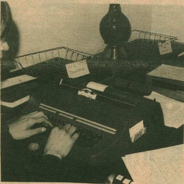
"Typesetting": After a story has been edited, the copy is typeset in 3 1/4" columns using an IBM Selectric Typesetter equipped with carbon tape.
