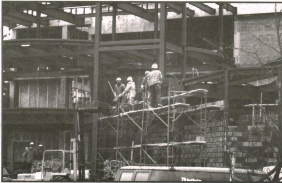
Workers move out the bricks in mid December.
