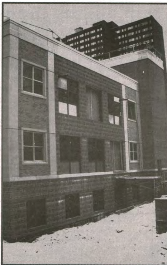
A view from the back of the building.
