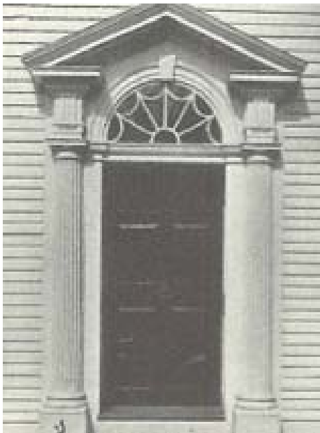
Figure 3-11: Federal doorway. Salem House, 1796. Available from: Abbott Lowell Cummings' Architecture in Early New England . 280
