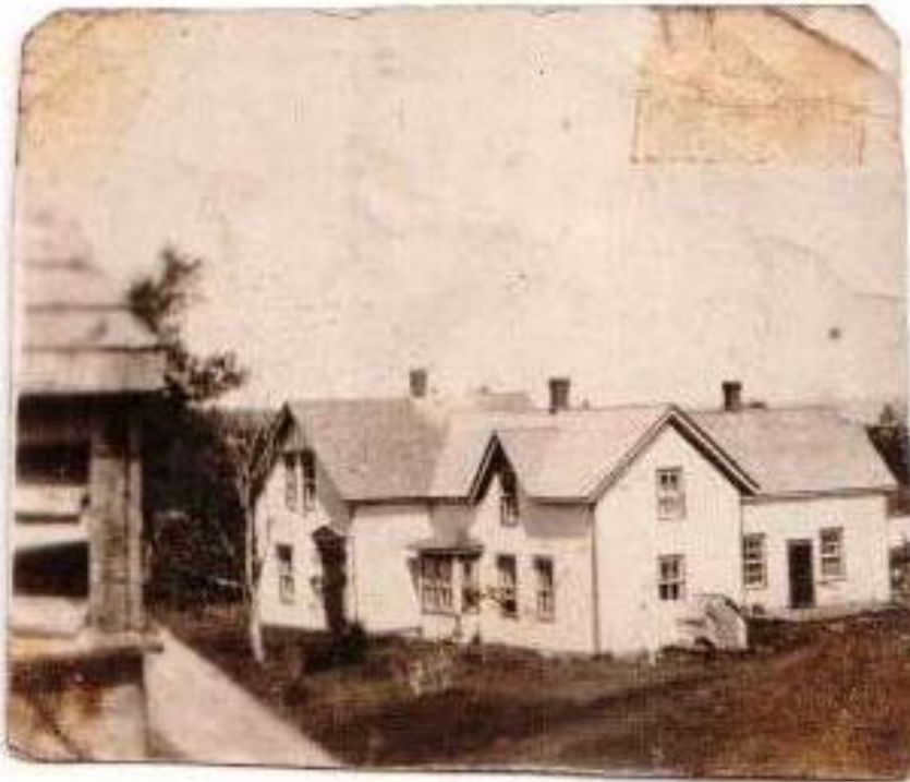
Figure 3-47: Configuration of the roofline of the Verge homestead after its pre-1900 relocation. Available from: Amber Hanrahan.
