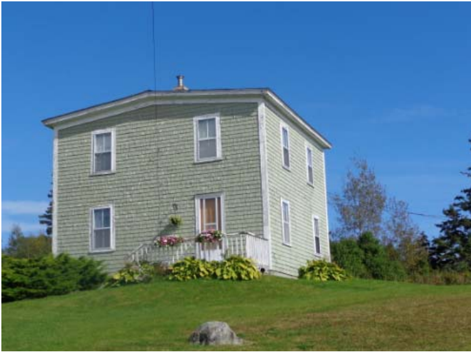
Figure 3-28: The residence of Marie Clancy and formerly her husband, Willis in Summerville, a hatch house, which was previously the home of Jessie MacKay and Annie Mackay Frellick. Available from: Amber Hanrahan. Photo date: 2013.
