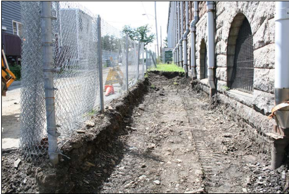
PLATE 10: Removal of topsoil along south side of building. Facing west.
