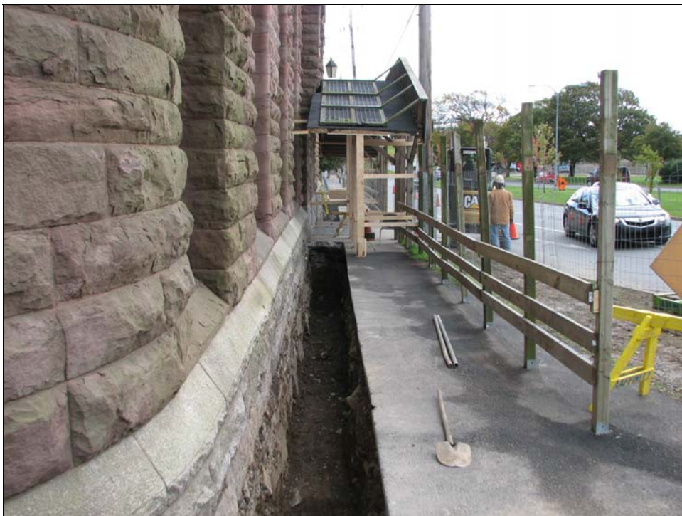
PLATE 12: Excavated trench along west side of building. Facing south.
