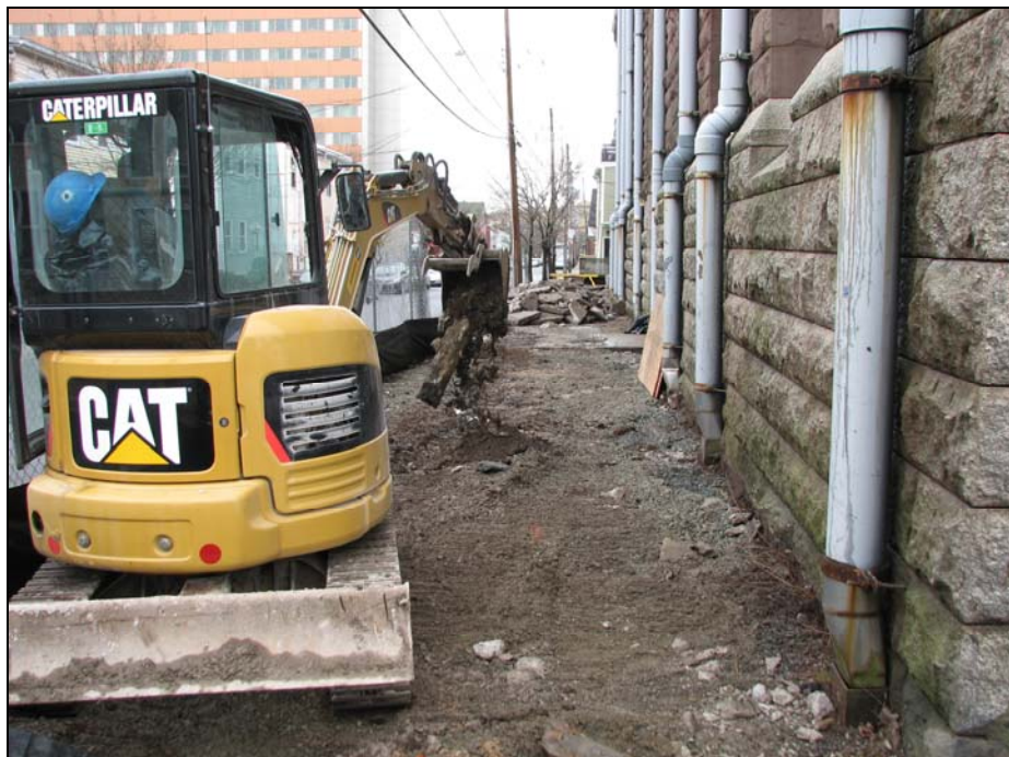
PLATE 8: Removal of sidewalk along east side of building. Facing south.
