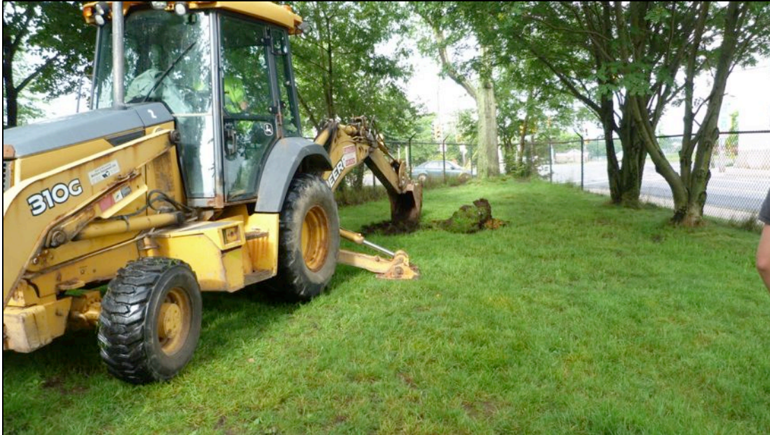
Plate 1: Looking west toward TP-01.
