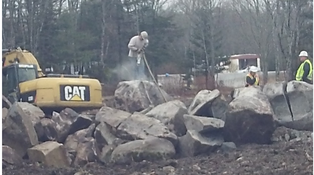
Breaking down the glacial erratics on the building site. (K. Cottreau-Robins, 2014)
