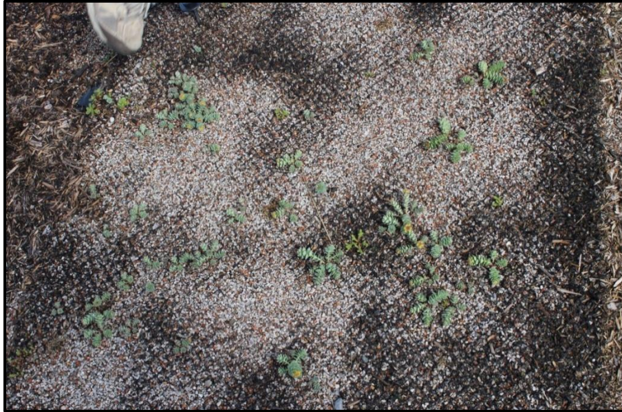
Figure 1: Rhodiola rosea growing on vegetated mat in Greenwich, Nova Scotia. Geotextile is visible where green roof substrate eroded away from the mat.
