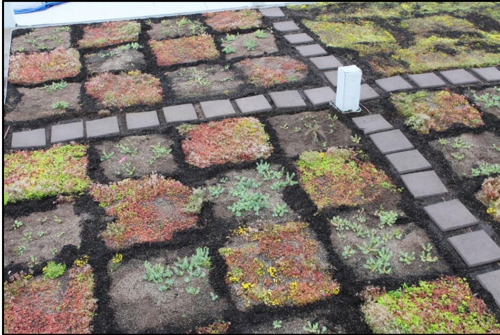
Figure 22: NSCC green roof plots immediately after installation on June 26, 2013 showing abundance of red Sedum album .
