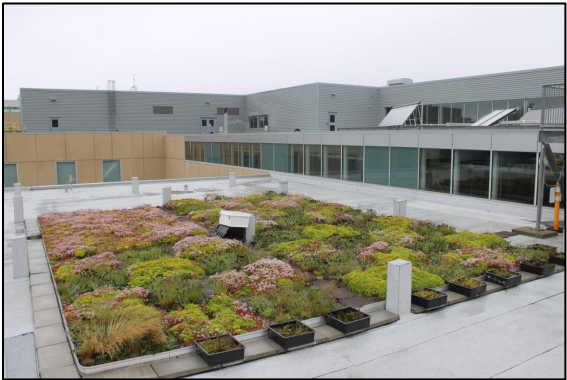
Figure 26: NSCC green roof in July 2014 at the end of the study period.
