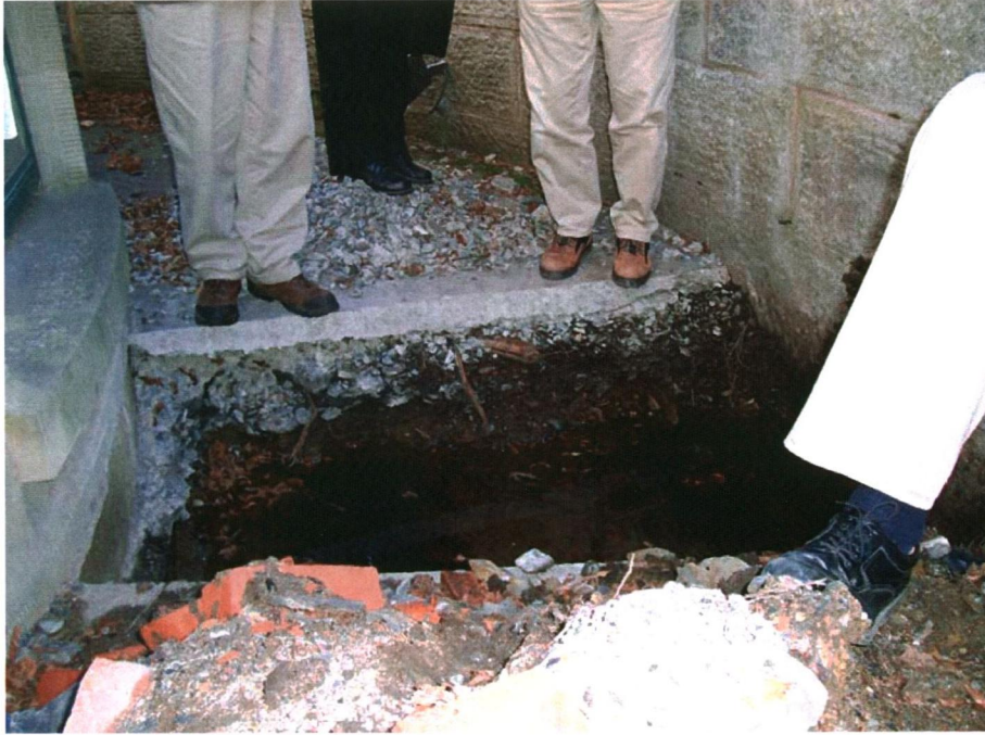
Plate 3: Removal of concrete and fill from south end of moat for initial inspection on 21 November 2006.
