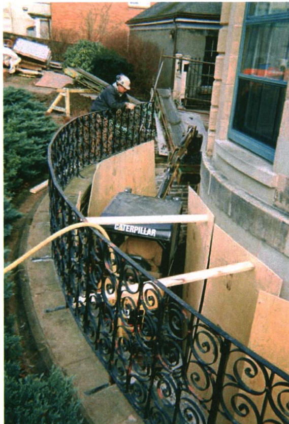
Plate 3: Removal of concrete and fill from south end of moat for initial inspection on 21 November 2006.
