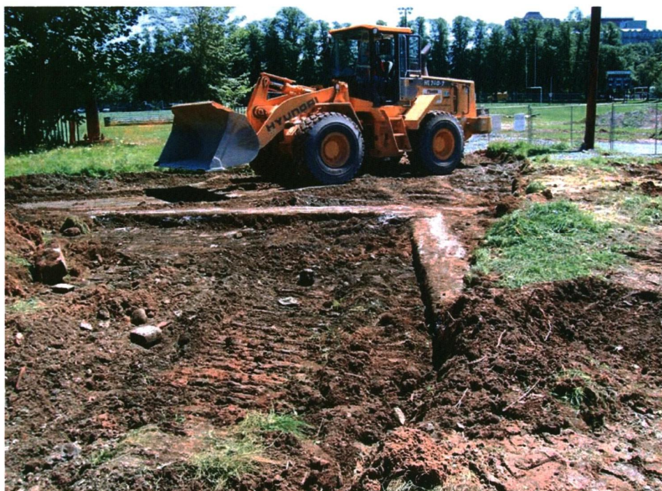
Plate 8: Exterior south wall (background) and interior partition wall (right) of the concrete footing to the west of the temporary paddock, looking south.
