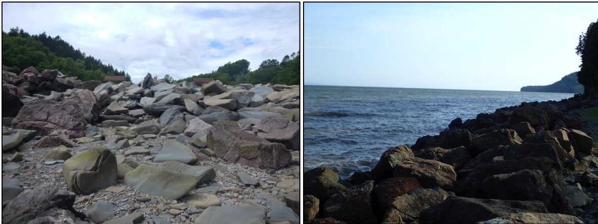
Figure 4.9. Intact riprap revetment at Cannontown Beach (L: June 2016, R: August 2016)
