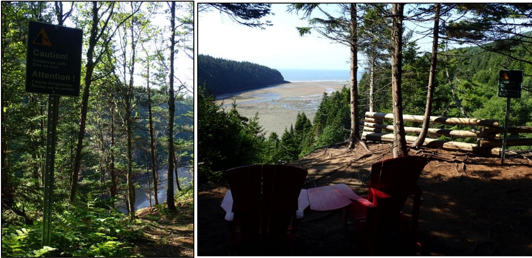
Figure 4.20. Signs warning visitors of dangerous cliffs below at various points along the Shiphaven trail overlooking the Point Wolfe estuary. There are trees falling to the bottom of the bluff just behind the fence in the photo on the right. (Photos taken August 2016)
