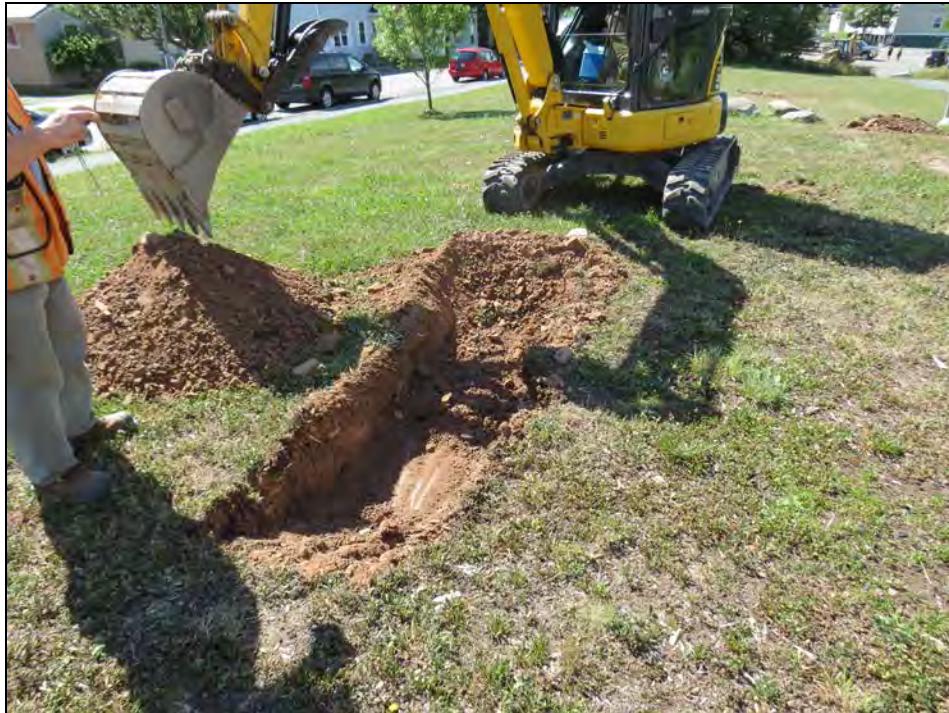
Plate 4: Profile of Test Pit 6; facing south. August 13, 2014.
