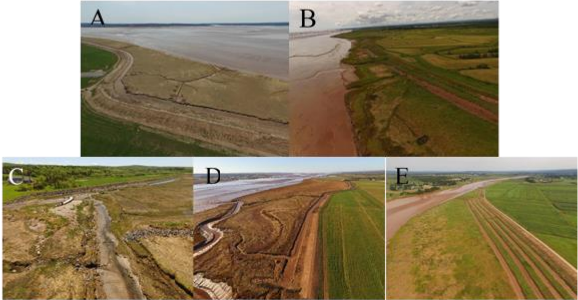
Figure 28: Borrow pits at A) Masstown West, B) Masstown East, C) Ryerson-Dugau, D) VDJ, and E) Lower Truro marshes.
