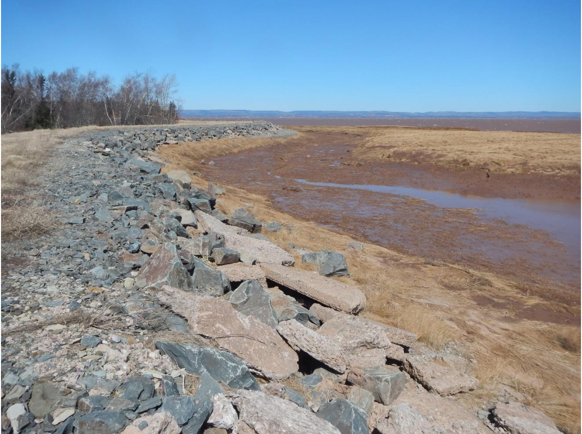
Figure 57: The borrow pit at NS024 Noel Shore (CBWES, 2019).
