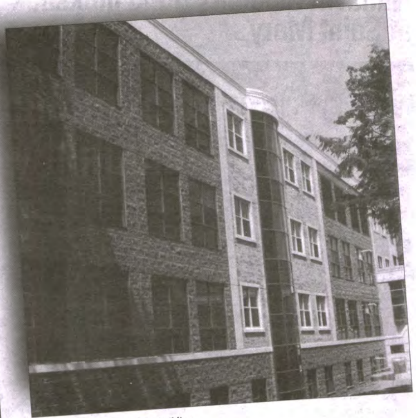
A view from the side of the building
