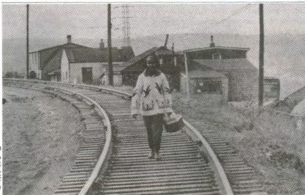
Along the railway tracks that sliced through the community.
