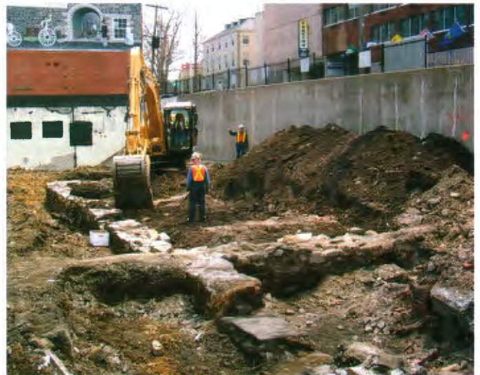
Steve Davis and Joe Cosgrove monitor mechanical excavation of stone foundations of row houses on Hollis Street.
