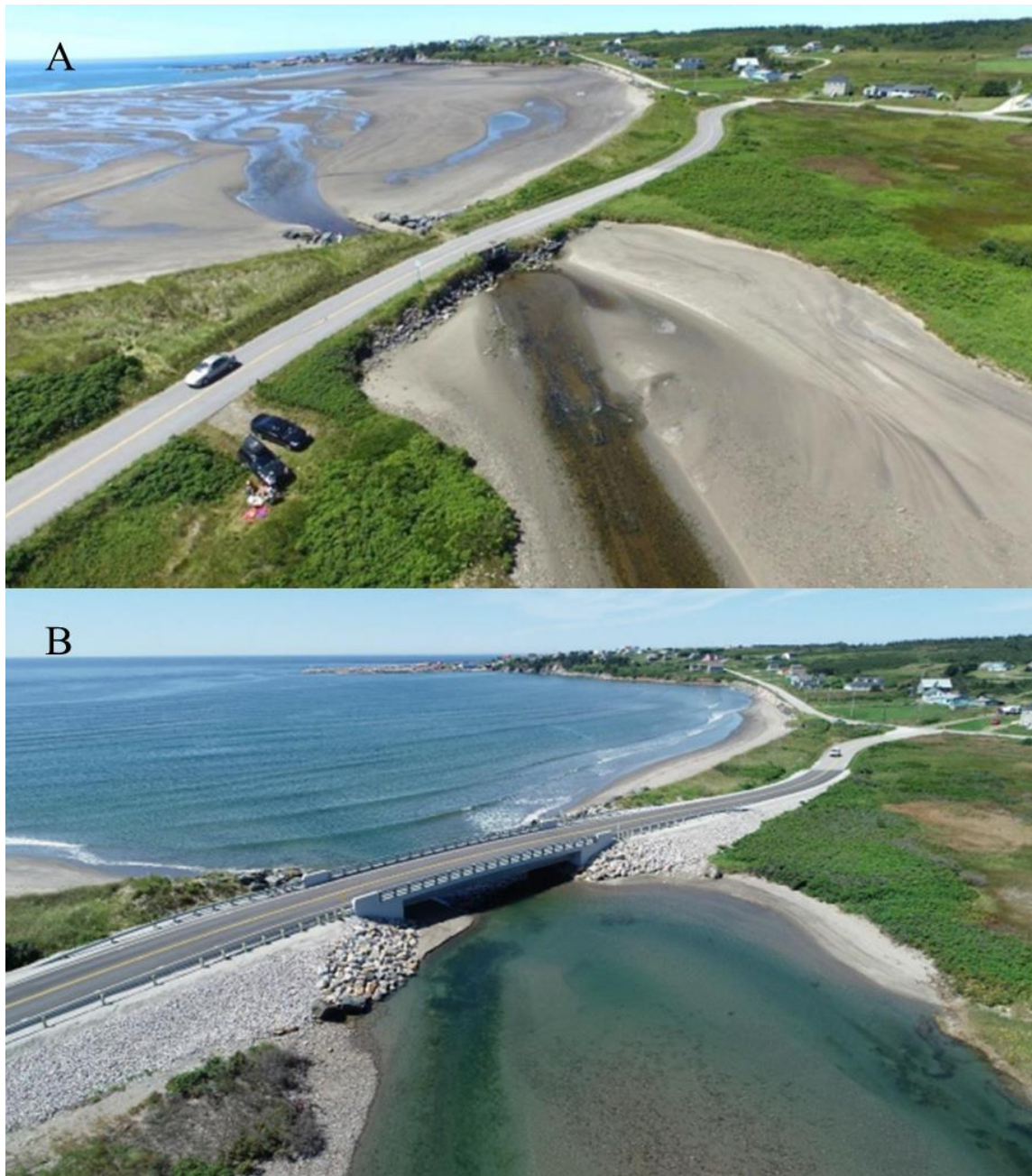
Figure 1.3. A) Pre-restoration (August 9, 2015) and B) post-restoration (August 15, 2019) aerial image of the primary tidal crossing on John Doucette Road at the Mavillette Tidal Wetland Restoration site. Photos by CBWES Inc.
