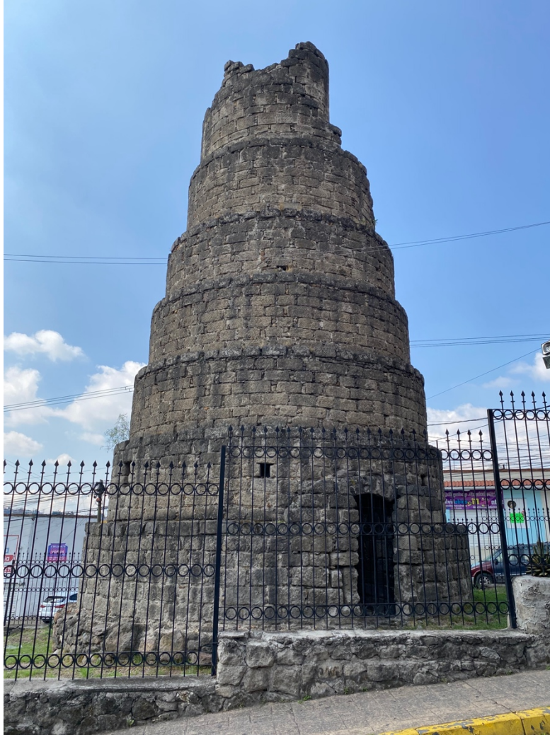
Vent tower in Los Remedios, State of Mexico. Photograph by Víctor Fuentes (02 July 2023).
