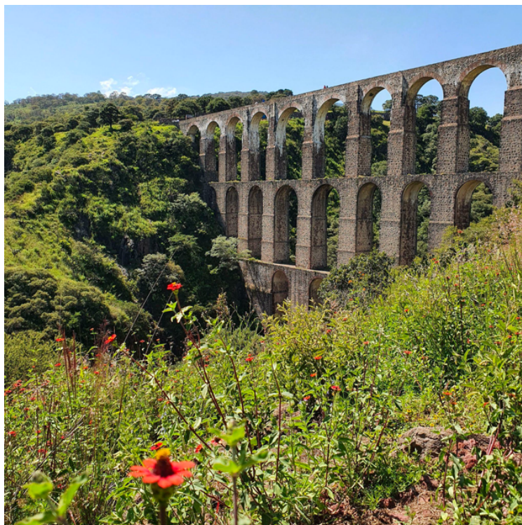
Aqueduct of Tepetzotlán. Photograph by Tania Fuentes, 2021.
