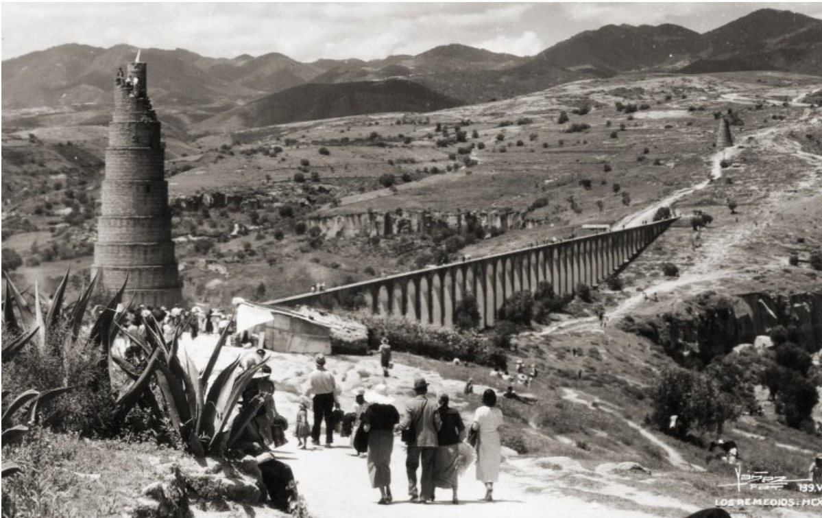
Vent towers Aqueduct of Los Remedios, ca. 1920s. Photograph by MexicoEnFotos , © Grupo Editorial Centli. MexicoEnFotos , https://www.mexicoenfotos.com/antiguas/mexico/naucalpan-de-juarez/acueducto-de-los-remedios-MX15430262340248/1 (Accessed 22 June 2023)
