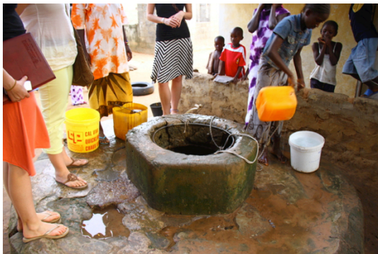
Figure 4.1 Unimproved Water Source (Uncovered Well)
