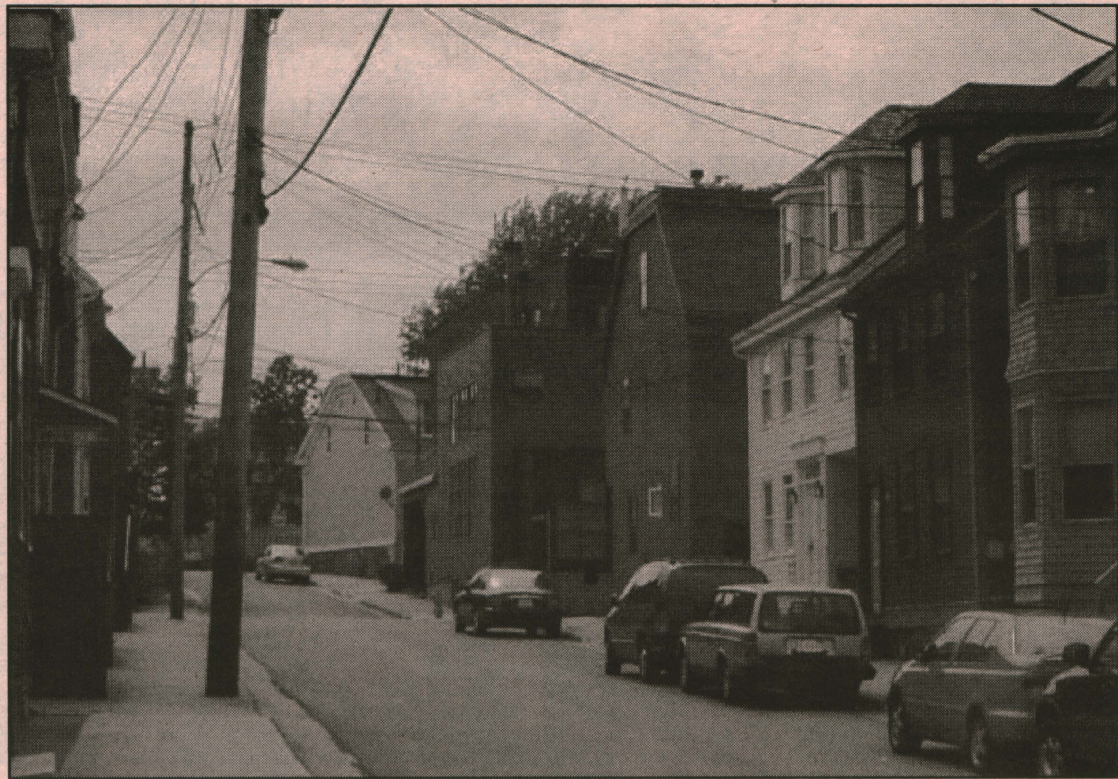
Falkland St. in the North End
