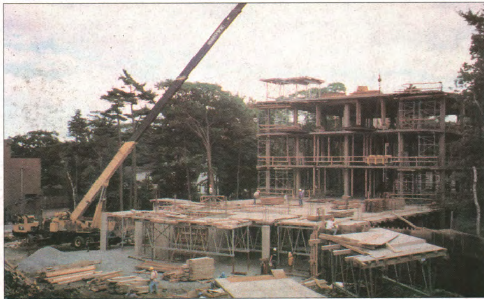
The building begins to branch out on August 23.
