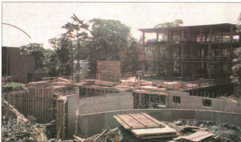
The building looks much larger during the first week of September.
