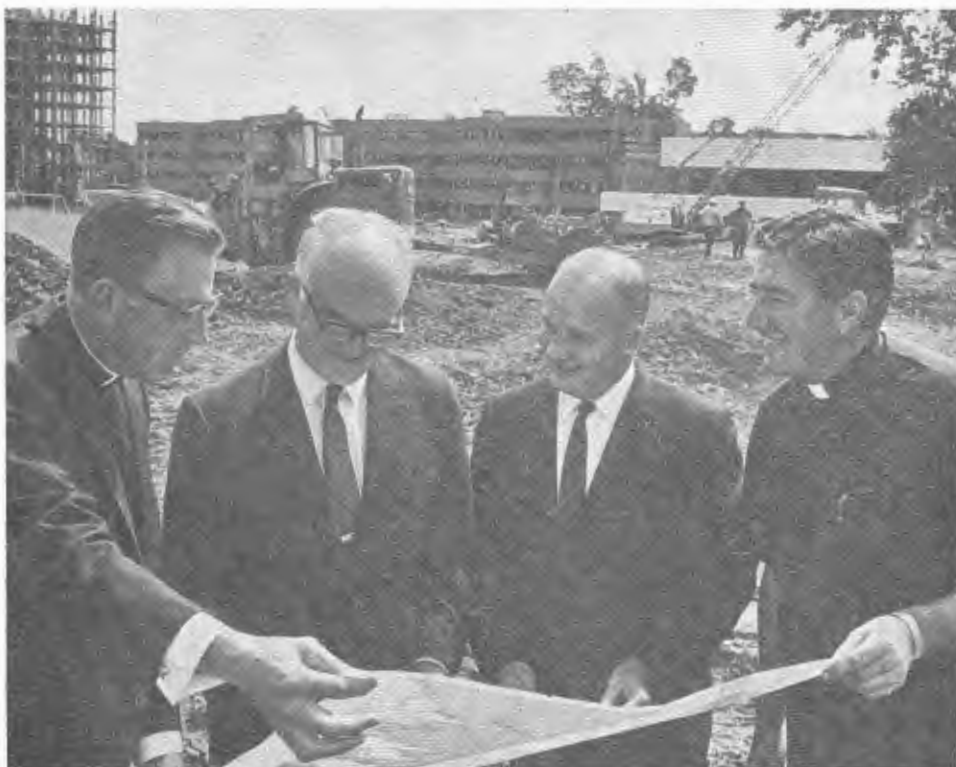
NEW STADIUM — Looking over plans on the site of the new 10,000 seat 1969 Summer Stadium are, left to right: Dr. H. J. Labelle , Mayor Allan O'Brien , Keith Lewis , general manager Summer Games and Rev. Robert MacDougall .
