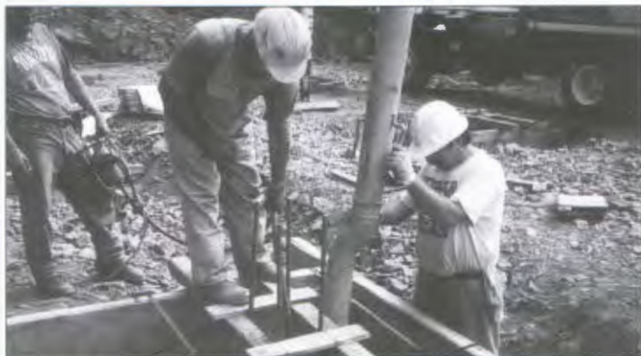
The first concrete being poured into the footing.
