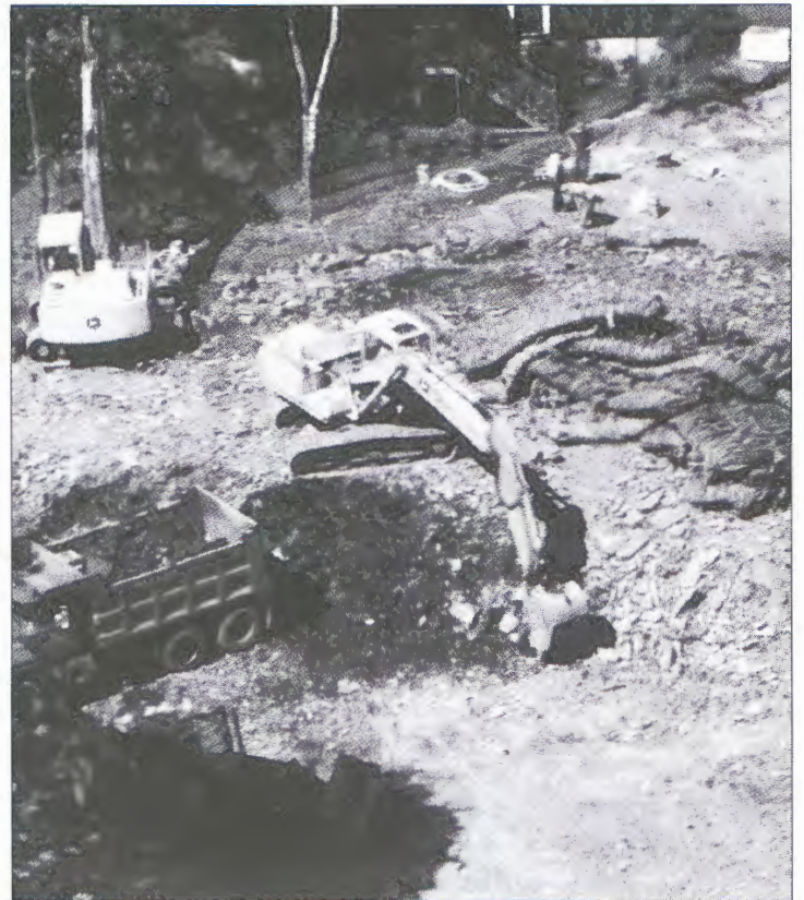
The excavation begins on June 18.
