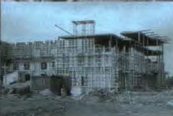
McNally Building under construction.
