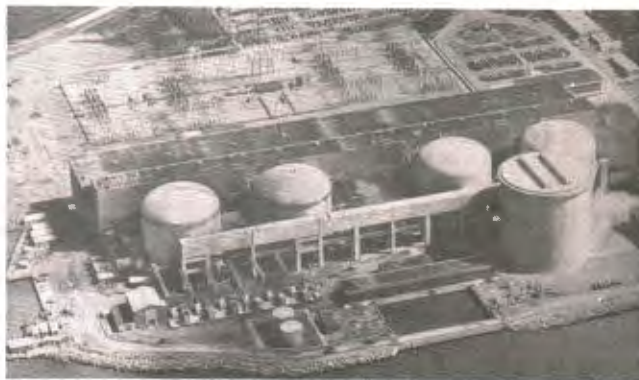
Ontario Hydro's Pickering Nuclear Generating Station has four reactors. The station, on the shore of Lake Ontario 20 miles east of downtown Toronto, is one of the largest nuclear power stations on the continent. Its four reactors are designed to produce more than 2,000,000 kilowatts of electricity at full power. All are now operating.
