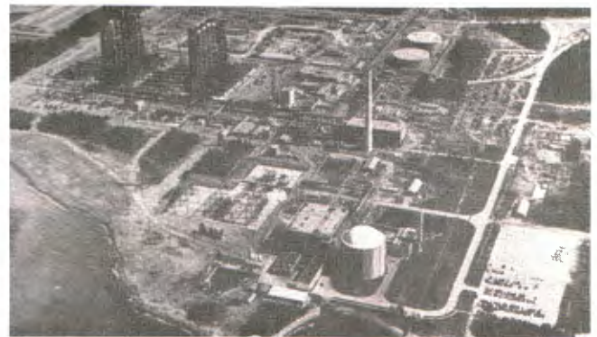
The Bruce Nuclear Power Development on the shore of Lake Huron in Bruce County, Ontario, is a complex incorporating Canada's first commercial size nuclear power plant, Douglas Point Nuclear Power Station, foreground, a heavy water plant which will produce 800 tons per year, under construction at left, and the Bruce Nuclear Power Station whose four reactors will produce 800,000 kilowatts each. The first is due to start up in 1975.
