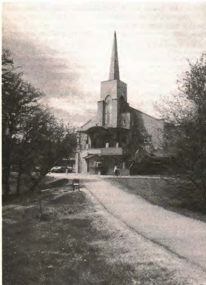
The back of the McNally Building with the steeple of the former Canadian Martyrs Church.
