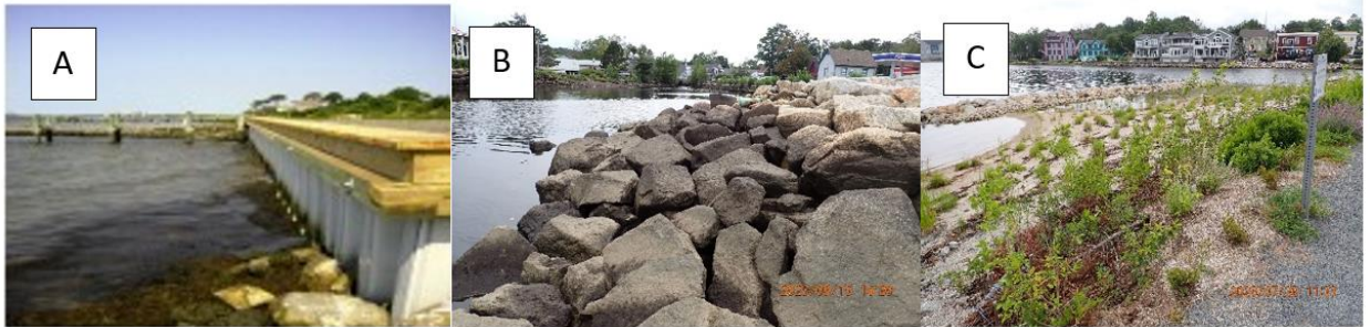
Figure 5. Types of Shorelines: A) Bulkhead, B) Riprap revetment, C) Sill (Modified from Figure 1. Gittman et al., 2014).
