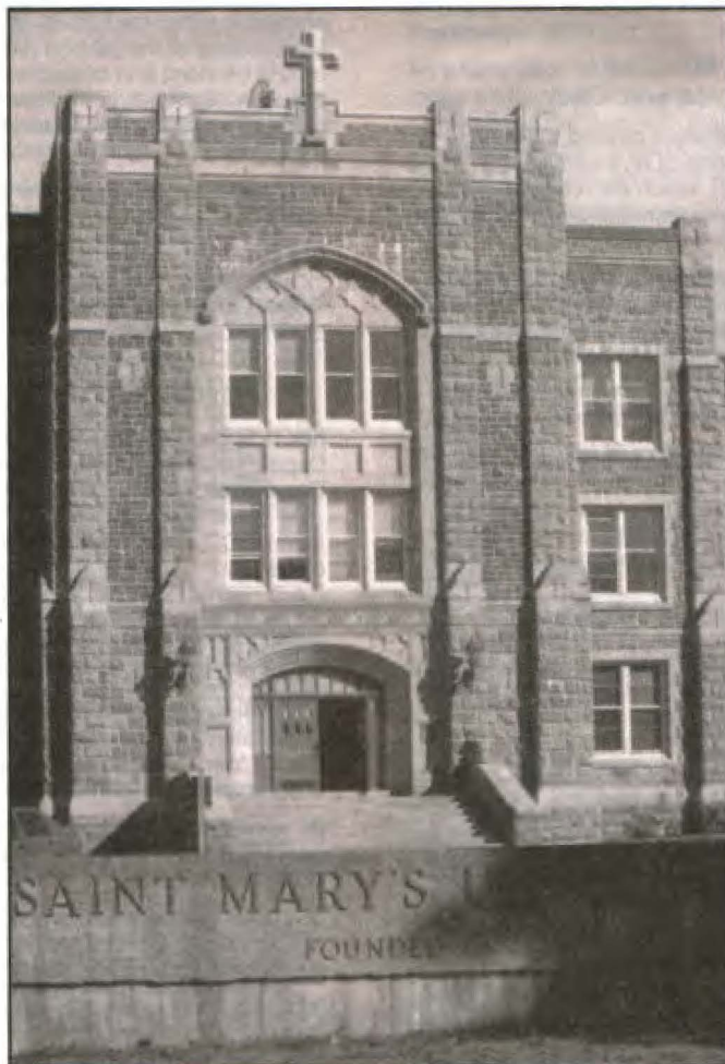
Main entrance of the McNally Building - the oldest building on campus.
