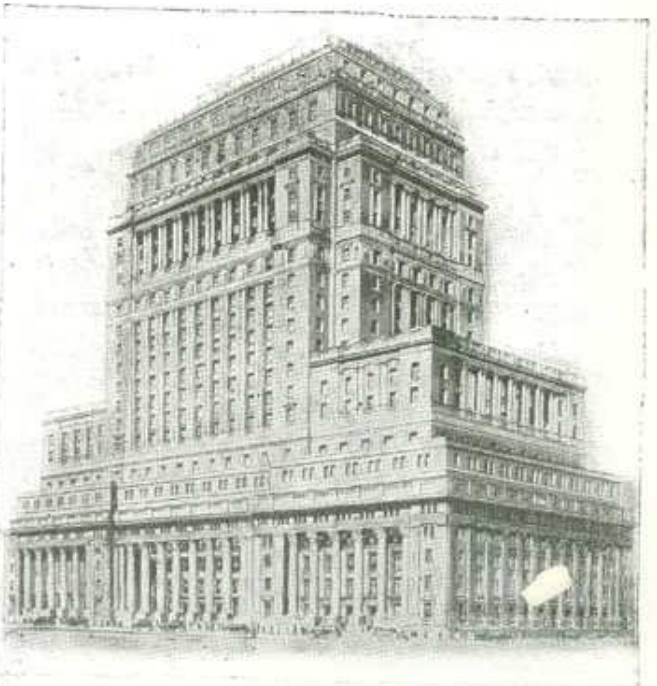
Sun Life Head Office Building, Montreal — entire exterior in Stanstead Granite from sidewalk to roof.
