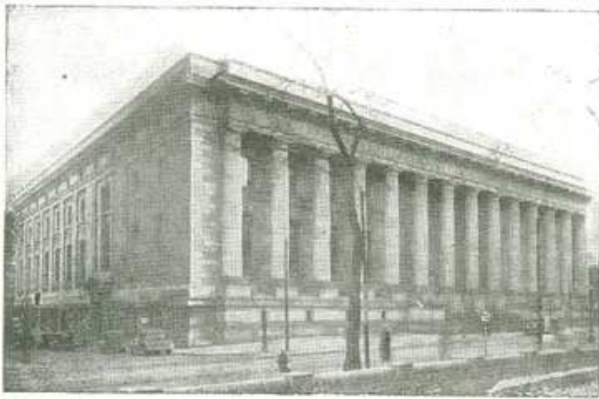
Montreal Court House—showing the imposing Stanstead Granite fluted columns on the broad facade.
