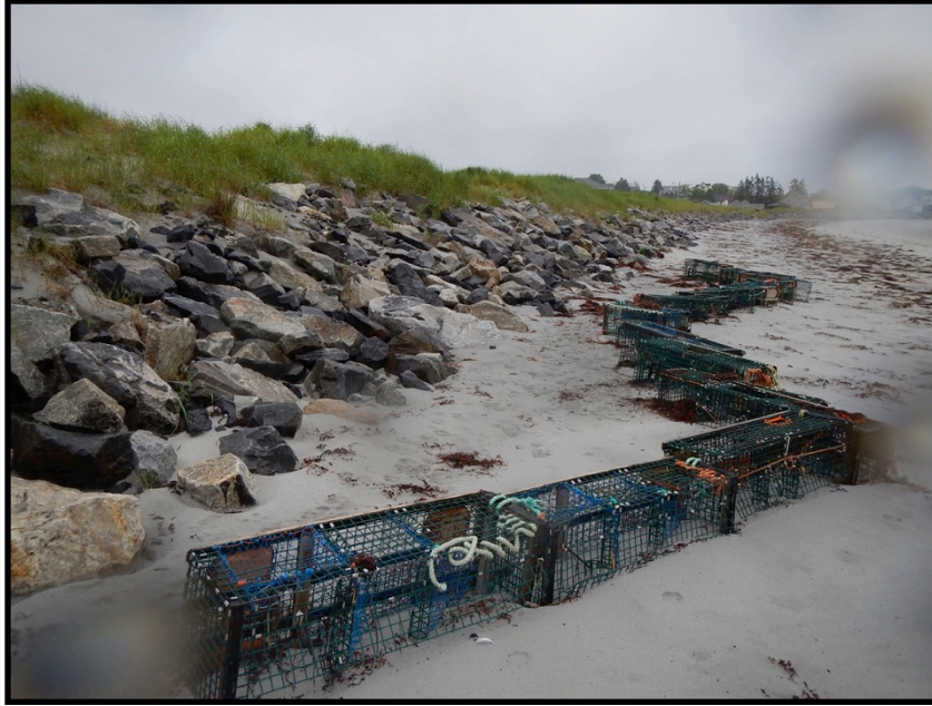
Figure 2.8 Lobster Traps used to Develop Foredune on Crescent Beach. (Photographer: Sam Page, 2013).
