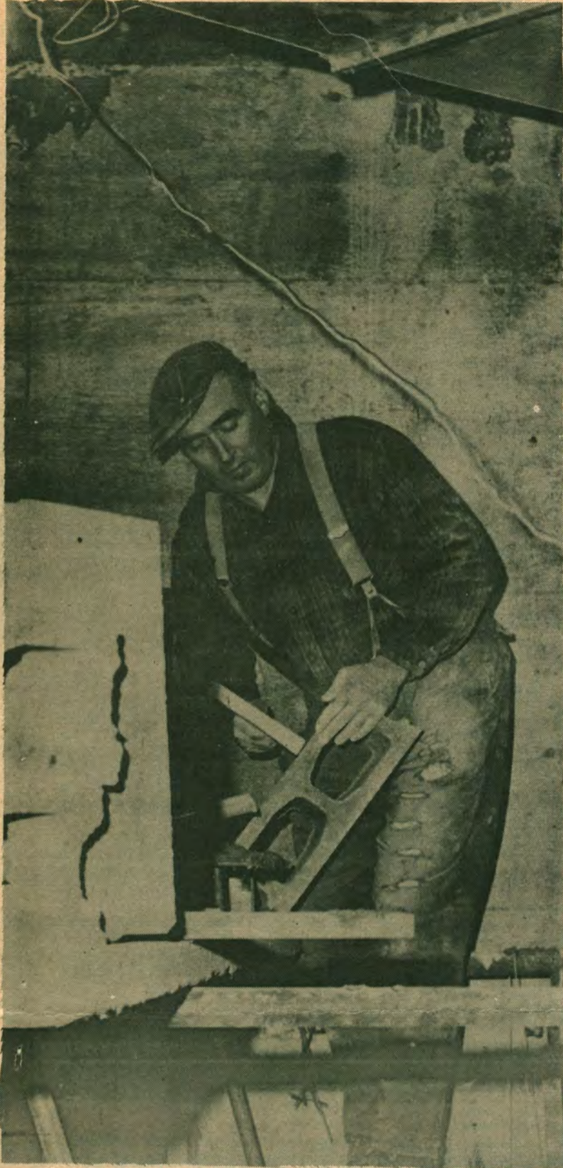
Apart from a few surprises in the plans, construction of the Centre is going on fairly well. Cement-block partitions have recently been completed all over the basement and ground floor will be completely partitioned shortly, giving one the feeling of being surrounded by telephone booths. The building should be ready for use during the 1967-68 term.
