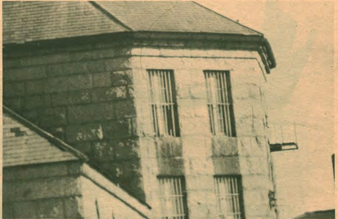
The century old Halifax Prison stands lonely and cold on a valuable piece of real estate in the extreme north end of the city.
