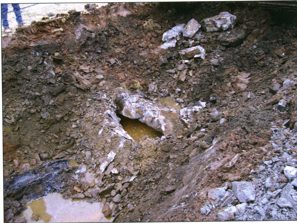
Plate 3: Top of the mortared stone culvert upon initial discovery. Backhoe has broken through the top of the feature.
