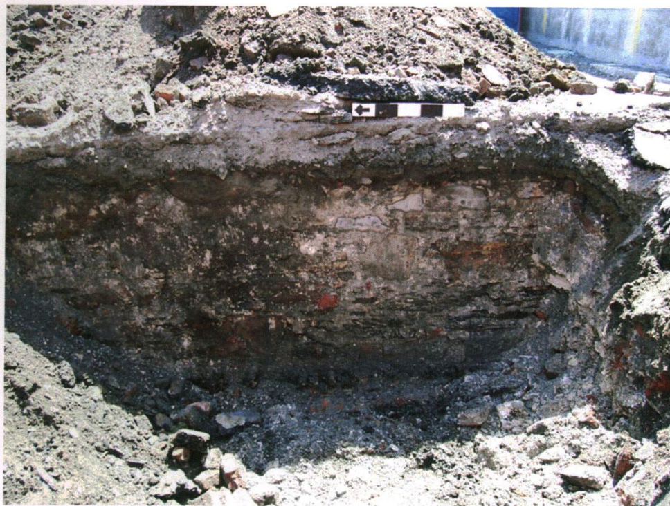
PLATE 2: North wall of Feature 3, unearthed during soils testing by Maritime Testing Limited.
