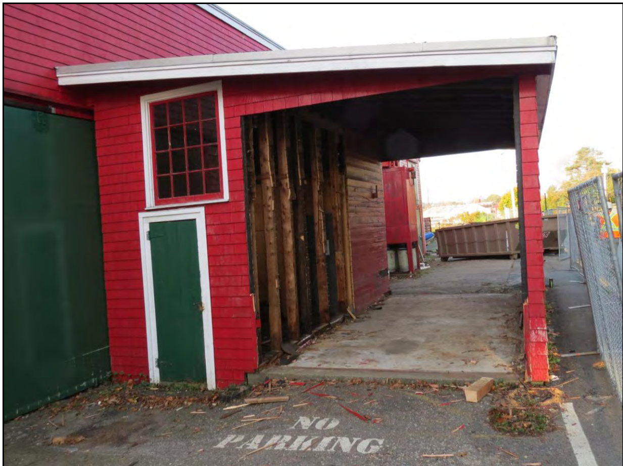
PLATE 25: Mechanical room during early stages of demolition; facing west; October 22, 2013.
