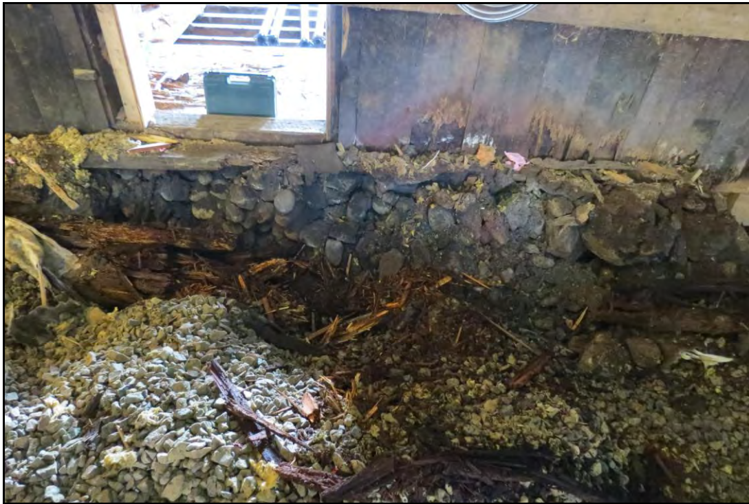
PLATE 14: South wall of the Inshore Fisheries Display Building resting on cobble fill; facing south; November 6, 2013.
