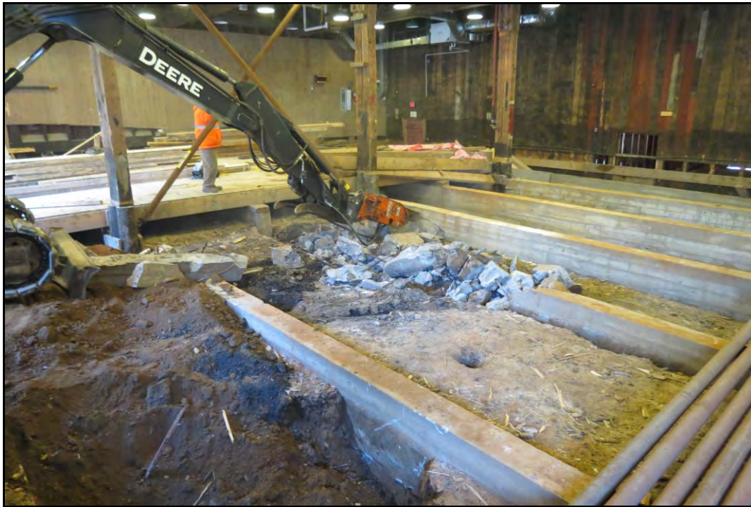
PLATE 4: Commencement of the break-up of concrete floor joists; facing southeast; October 22, 2013.
