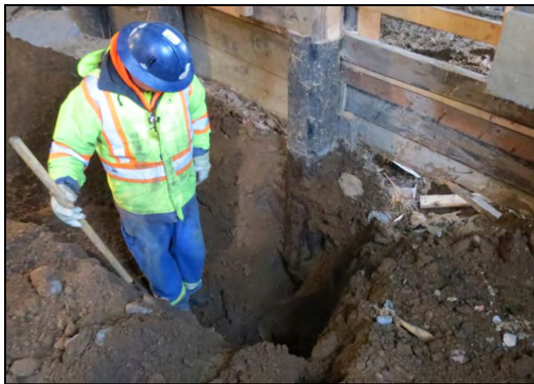
PLATE 11: Test excavation of support post along west wall of the Inshore Fisheries Display Building; November 5, 2013.
