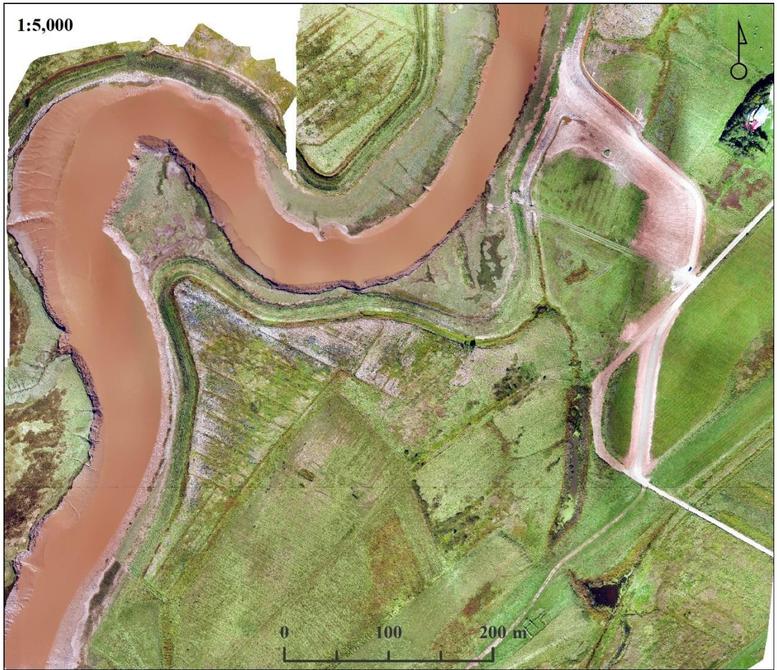
Figure 2.5: RPAS orthomosaic of Converse collected on September 24, 2018 (RPA model: DJI Phantom 3 Professional; flight altitude: 90 m). The construction on the new dyke and the road are finished by using material from the borrow pits. The survey took place for the pre-breach classification analysis. (Credit: Akyol, R., Saint Mary's University)
