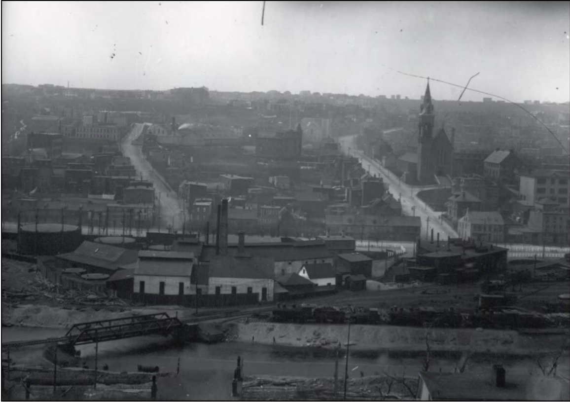
Plate 3: View of West End St. John's, 1914, looking northwest across the Waterford River Bridge. 141
