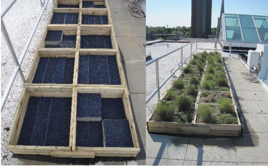
Figure 3. Construction and placement of the soil depth heterogeneity experiment. The image on the left depicts the planter boxes before substrate and vegetation was added. The image on the right depicts the planter boxes after planting.
