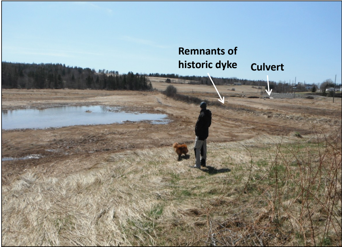
Figure 2. 2 Northern section of Cheverie Creek Restoration Site displaying a portion of the historic dyke in relation to the culvert (C.Skinner, 2014).
