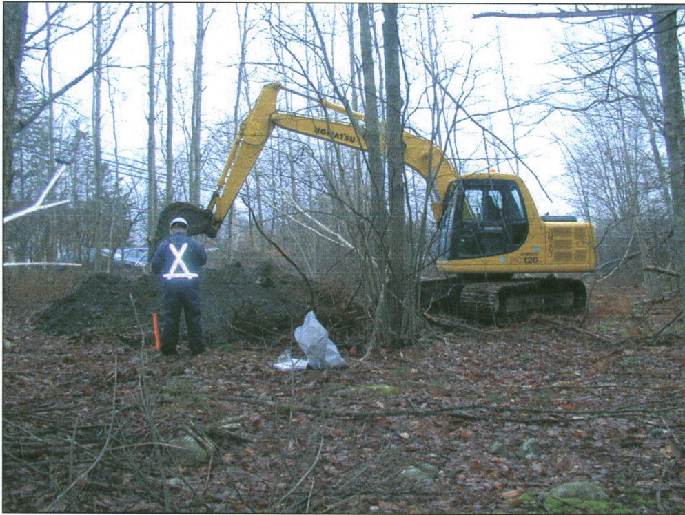
Plate 4.0.1: Geotechnical testing, TP4 (1 December 2004).
