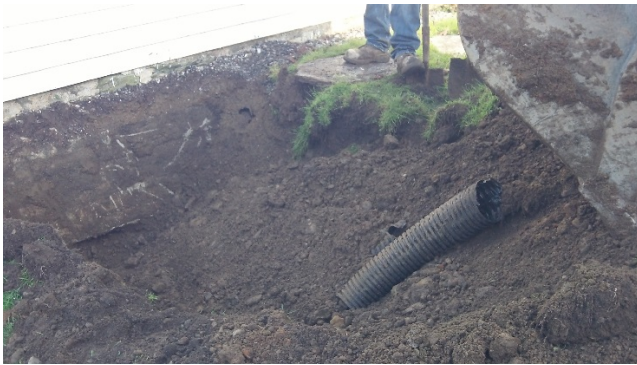
Foundation partially exposed in Area A. See modern plastic pipe remnants amongst the fill.
