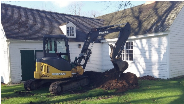
Excavation Area B located at the rear of Perkins House in the western area.
