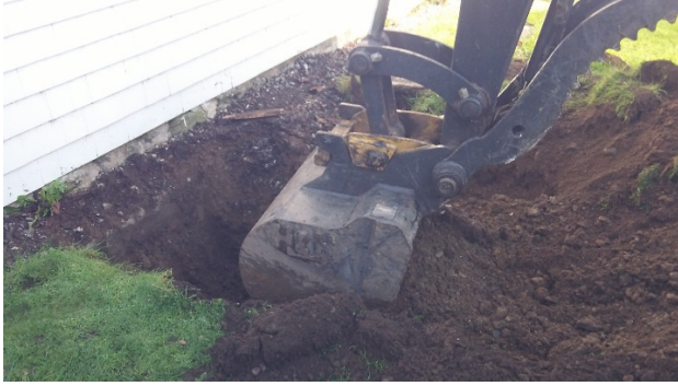
Excavation underway at Area A. (K. Cottreau-Robins, 2014)
