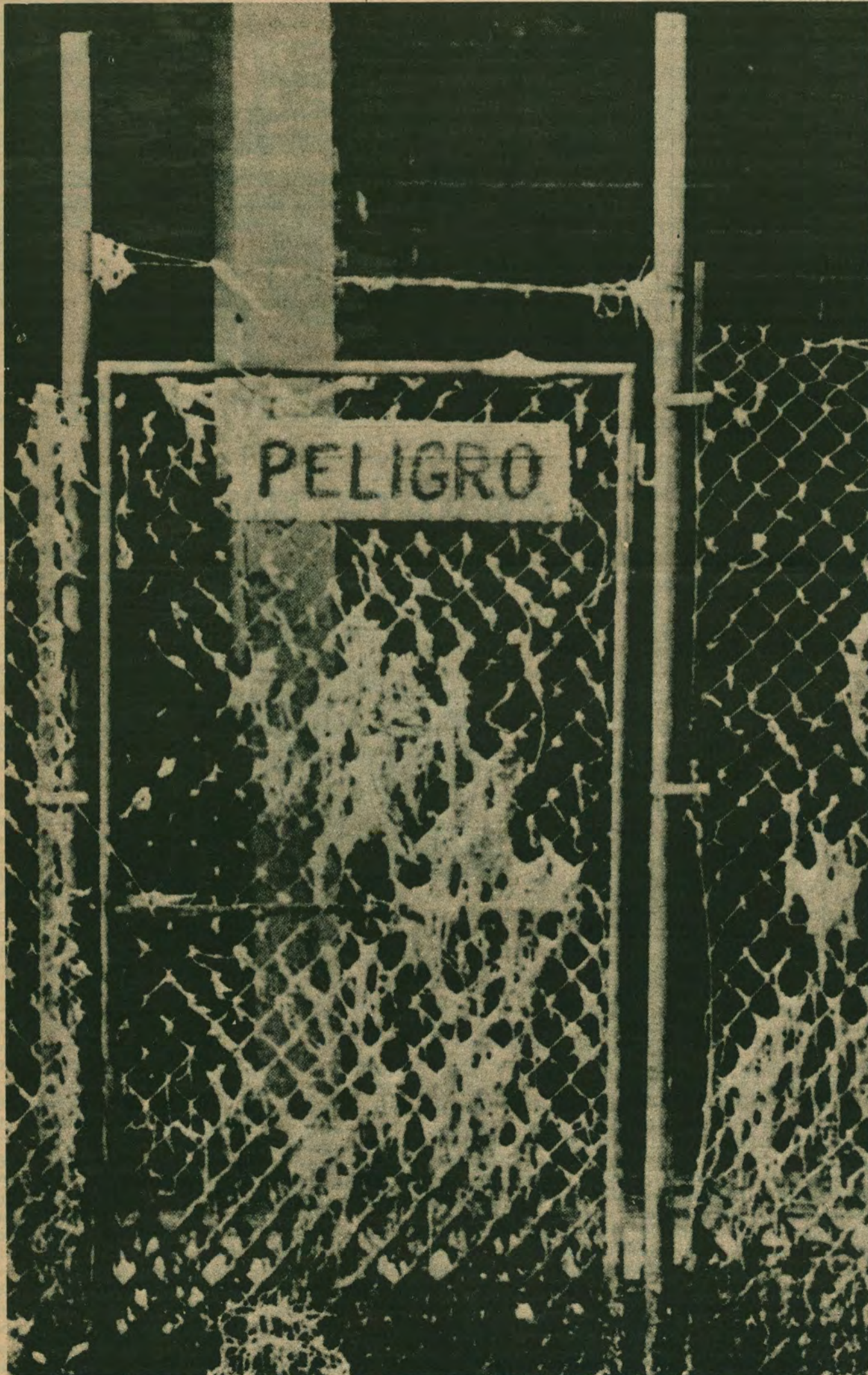
The sign says, "Danger". But the absentee owners of the Amatex plant in Agua Prieta do nothing to curb the flow of asbestos fibres that cling to the fences, the streets and the people of this northern Mexican town.
