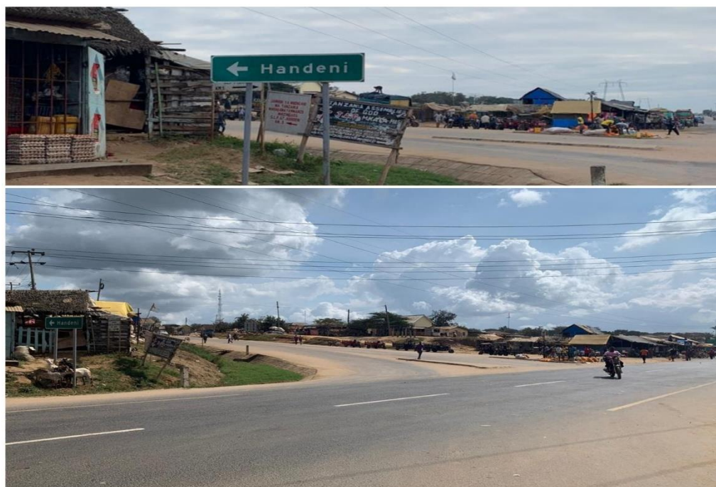
Image 7: Tarmac road connecting Handeni to a major highway
