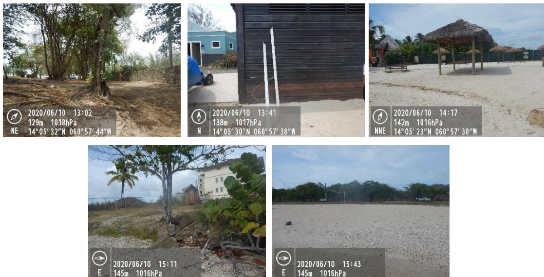
Figure 5.6 Pigeon Island Causeway profile vertical markers A (top left), B (top middle), C (top right) D (bottom left), E (bottom right)
