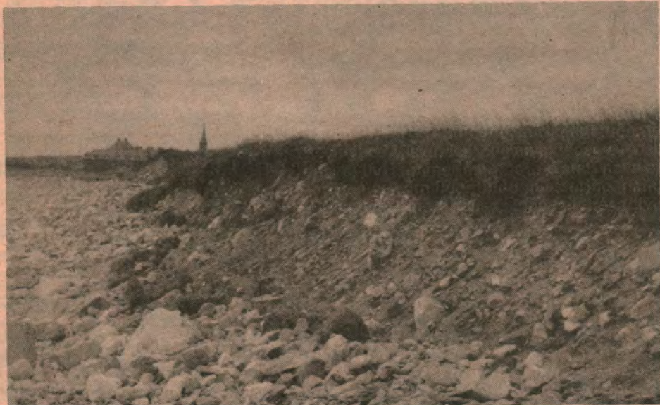
Eroding shoreline near Fortress Louisbourg, Nova Scotia
